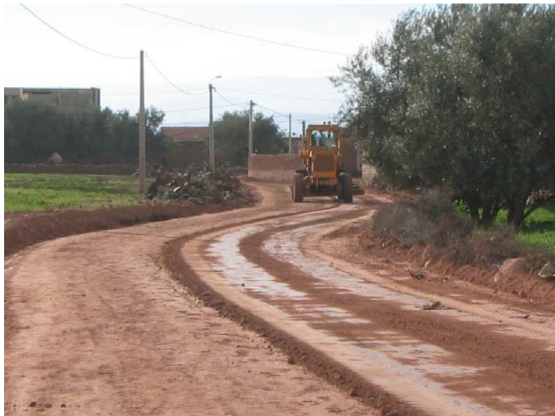
Final shaping of the road
