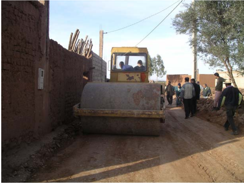
Compactor, compacting the road
