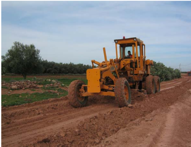
Grader blading material into a windrow
