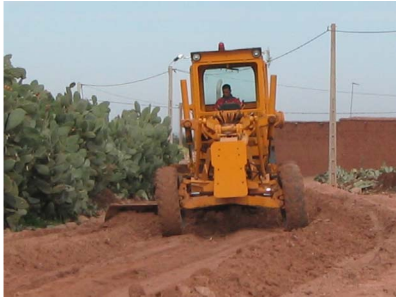
Grader mixing RAPIDroads y windrowing the material side to side
