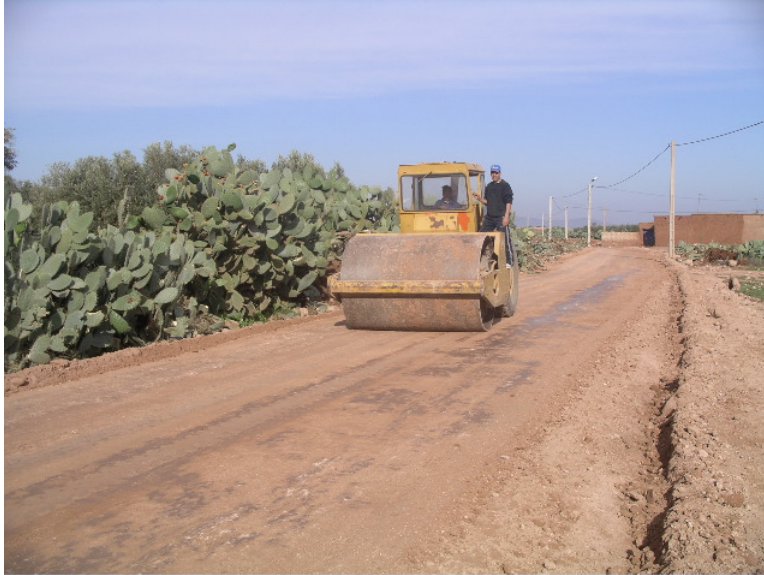
Final compaction of the road
