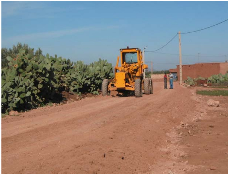
Grader spreading material and shaping the road
