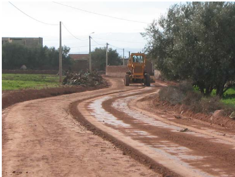
Final shaping of the road
