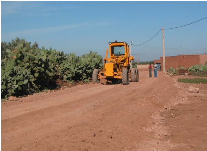
Grader spreading material and shaping the road
