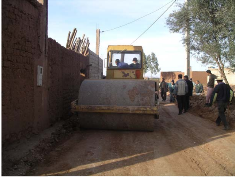
Compactor, compacting the road
