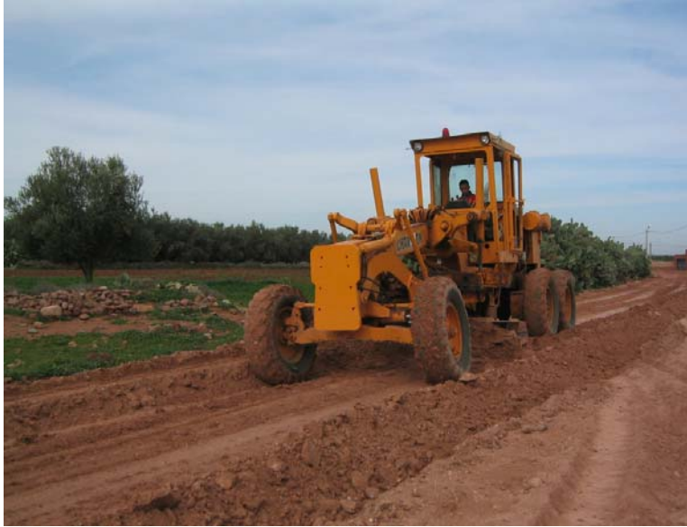
Grader blading material into a windrow
