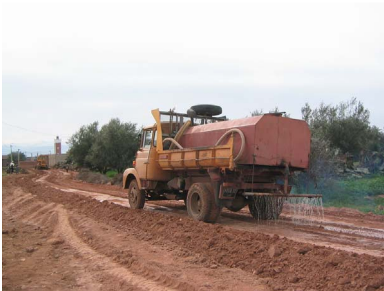
Water truck adding RAPIDroads to windrow materials and sub base
