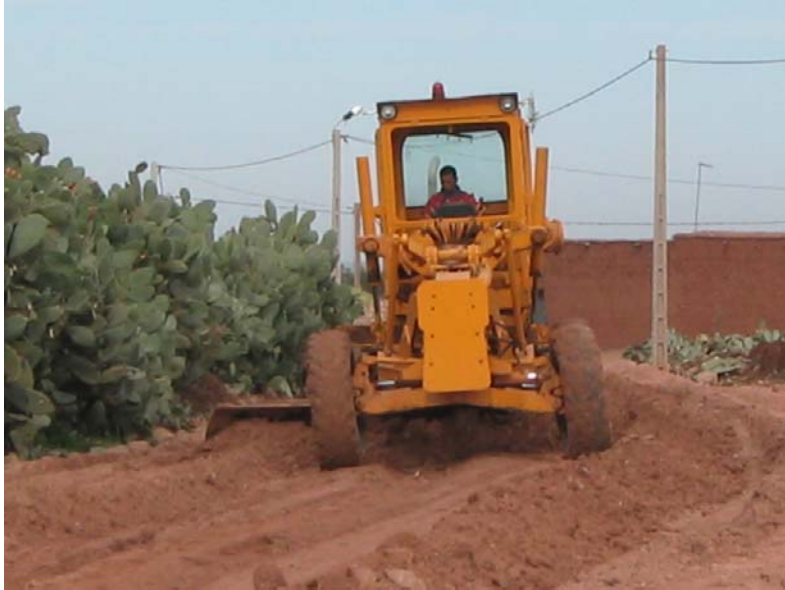
Grader mixing RAPIDroads by windrowing the material side to side
